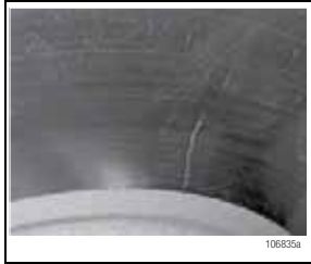
Acceptable Crack FIGURE 109
